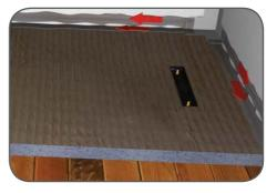
Step 11 Where the shower tray meets the wall apply a thin layer of Pro-SEAL tape sealer to the shower area and the adjoining wall approximately 60mm wide on both.
