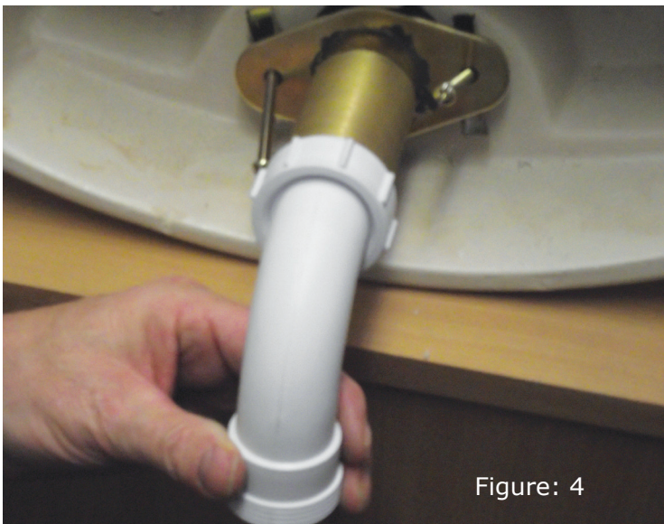
Figure 4: Fasten waste connector on to waste outlet.
