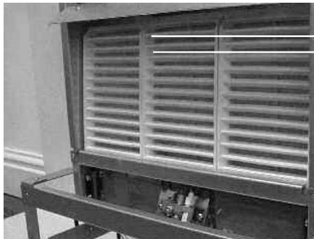
Smoke match position approx. 5mm below and inside the front edge of the combustion chamber lid.
