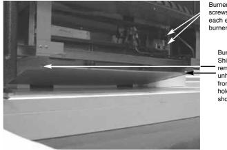
Burner retaining screws (2 off at each end of burner)
