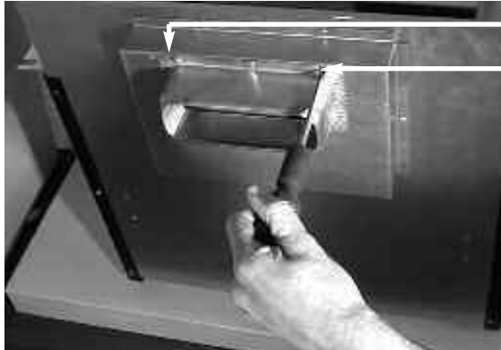
4 off Flue Spigot Fixing screws
