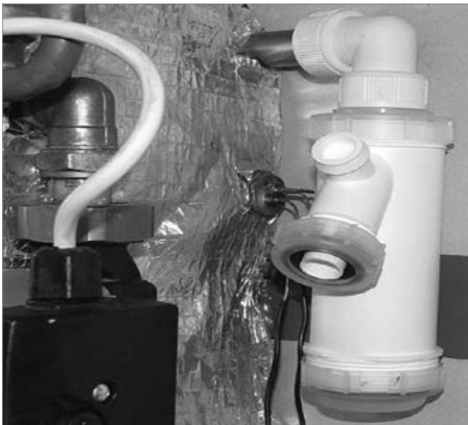
Figure 6-2: Condensate trap location
