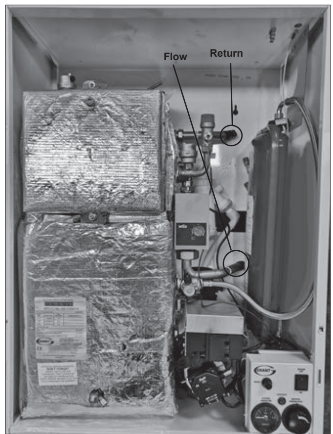
Figure 5-2: System boiler flow and return connections
