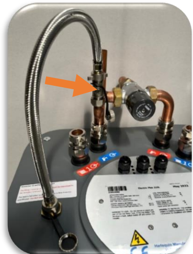
Figure 5 Filling loop connected
