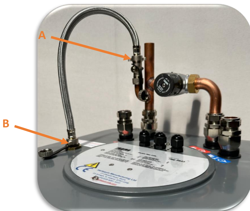
Figure 14 Hot and cold-water connections
