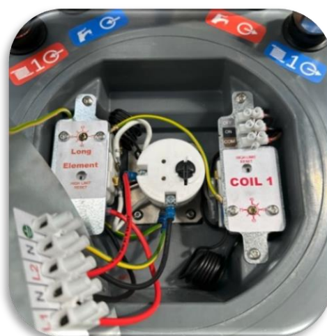
Figure 3 Immersion heater and thermostat compartment
