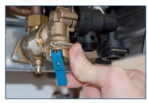
Whenever the system needs to be re-pressurised, the blue lever is simply pulled down until the correct pressure is achieved.
